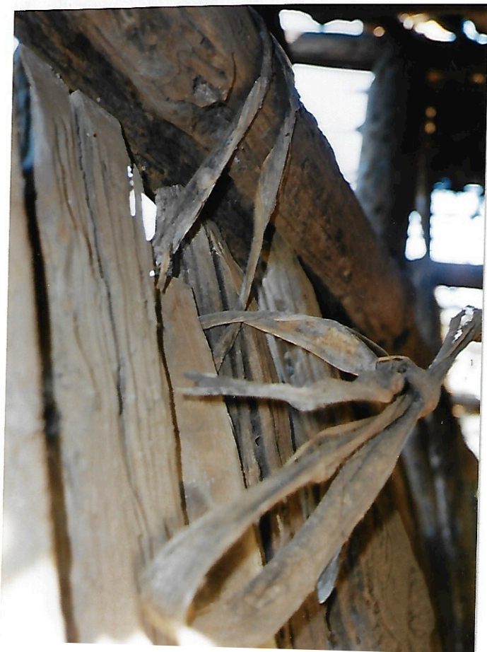
On the left a wall of a cow stable there is a groove in the upper beam to hold the planks. On the right a fence for the pig Stable. All pictures are taken in Dupi.
