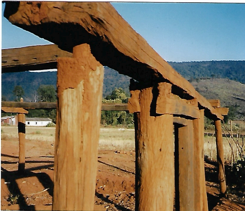
An old frame of a house in the village Dupi. It is typical construction of a house out of Sal wood. In between the wooden construction has been a mud wall.
