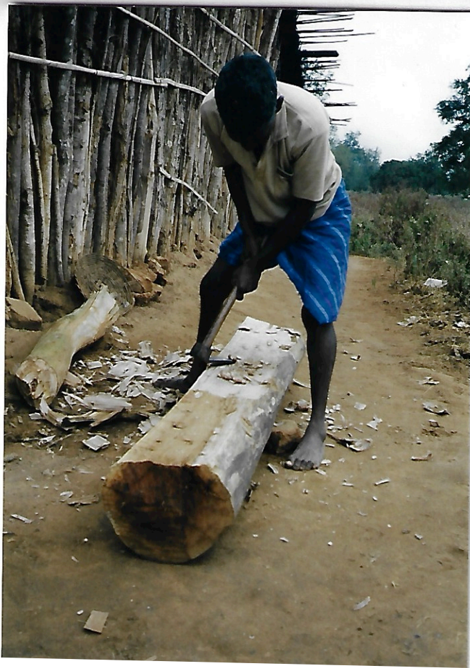
Here two handled adze used to prepare a beam for mortar. This beam with a couple of holes will be in the floor of the house. All pictures are taken in Telengapadar.
