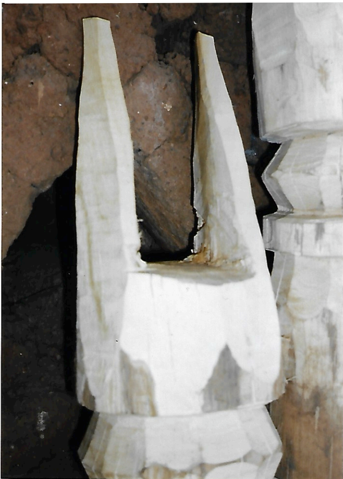
Jatra Kudi Munda prepared posts for the rituel house. If possible this posts are made of sal- wood or from Damana wood ( Grewia tiliaefolia Vahl. )
