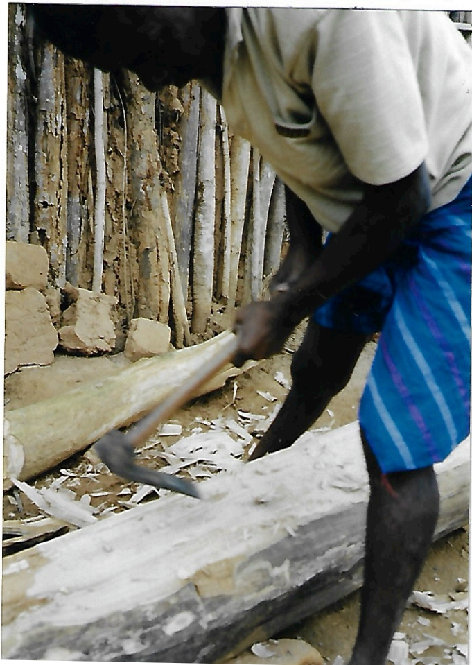
Here two handled adze used to prepare a beam for mortar. This beam with a couple of holes will be in the floor of the house. All pictures are taken in Telengapadar.
