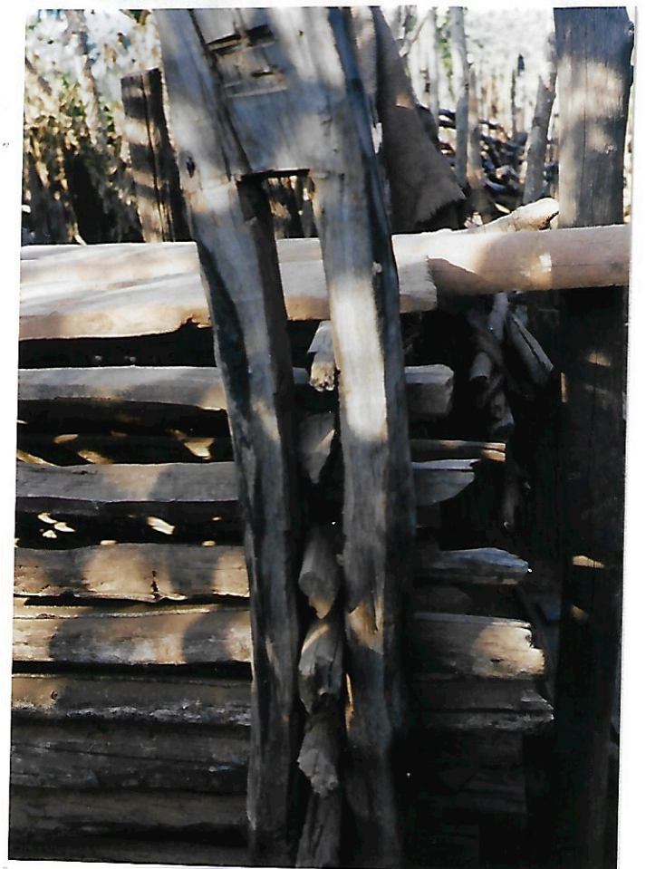
On the left a wall of a cow stable there is a groove in the upper beam to hold the planks. On the right a fence for the pig Stable. All pictures are taken in Dupi.
