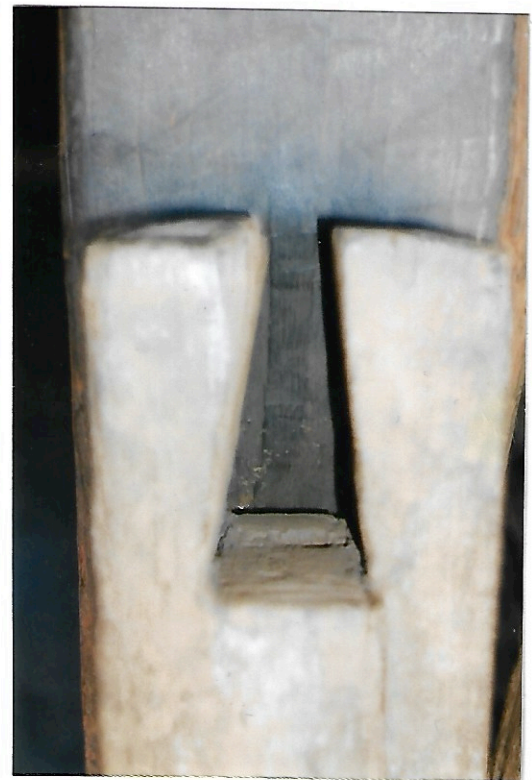
An old frame of a house in the village Dupi. It is typical construction of a house out of Sal wood. In between the wooden construction has been a mud wall.
