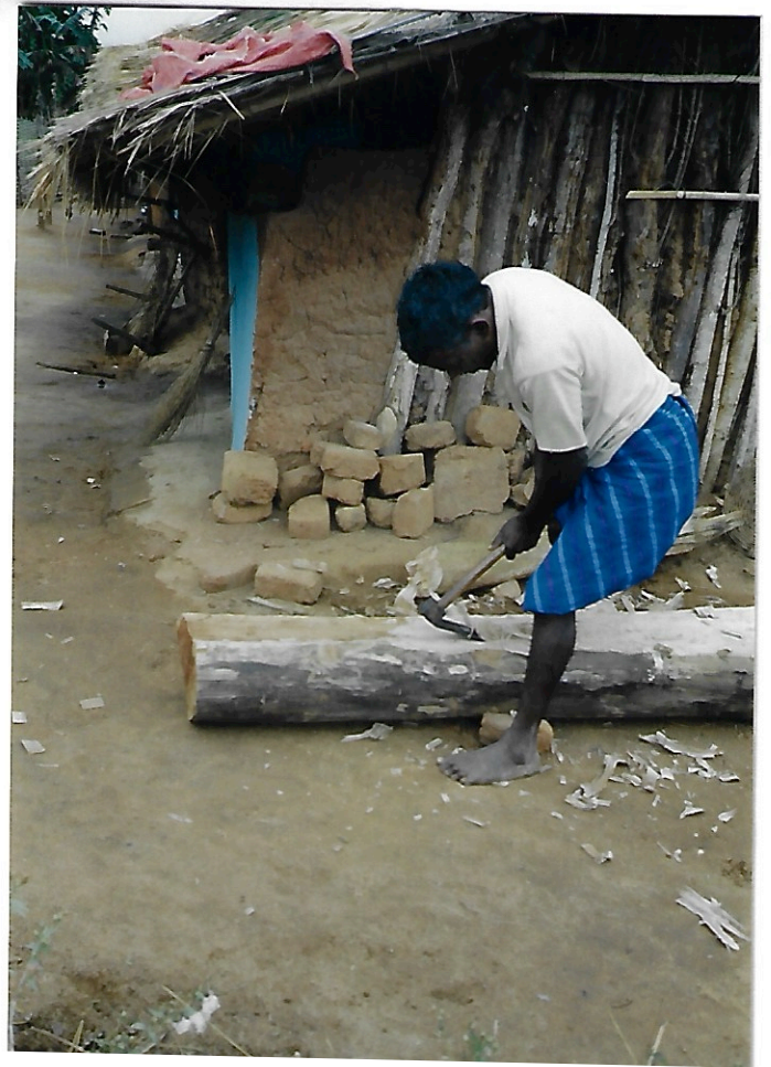
Here two handled adze used to prepare a beam for mortar. This beam with a couple of holes will be in the floor of the house. All pictures are taken in Telengapadar.
