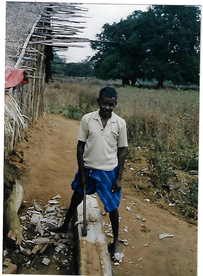
Here two handled adze used to prepare a beam for mortar. This beam with a couple of holes will be in the floor of the house. All pictures are taken in Telengapadar.
